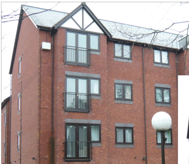
Examples of contemporary and traditional juliette style balconies in the immediate surrounding area ( along Park Avenue )
